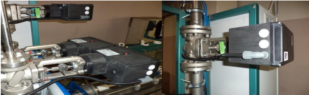
Figure 16 - Regulator Valves
